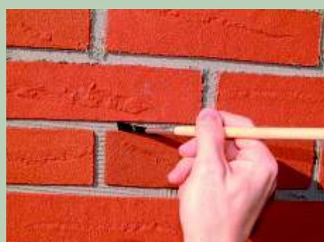
Smooth joints with a damp brush.
