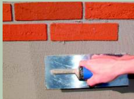
Apply Flexi-Brick™ mortar/adhesive.
