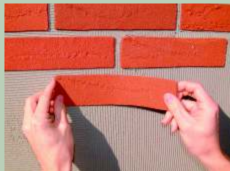
Press bricks firmly into mortar.
